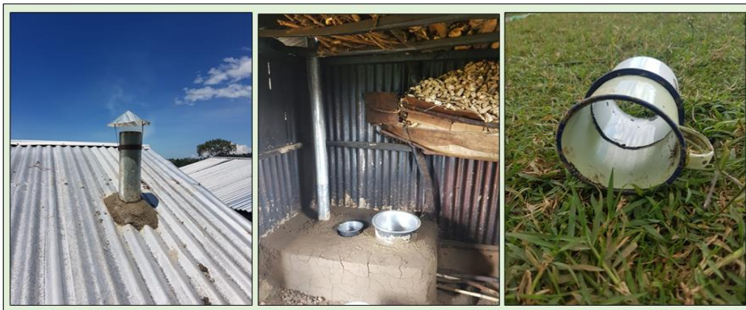
Figure 2: Left - Views of the chimney outside/inside the house / Right - Construction guide for the connecting duct between the two pots (Authors, 2021)
